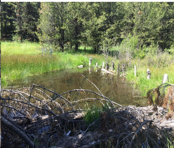
Looking downstream at an ABD. Small tree stems and limbs are woven among wood posts driven in the stream channel to function like beaver dams.
